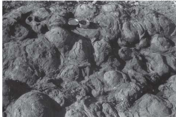
Fig.6.4 : Exfoliation (Flaking) and granular disintegration
